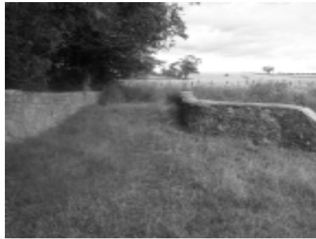
The eastern – and older? – bridge
